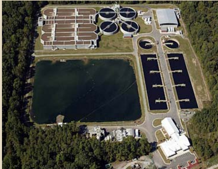
A Local Waste Water Plant
